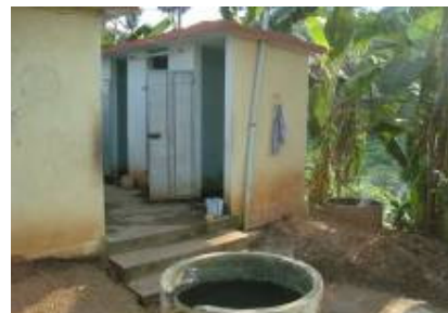
Total Set of Facilities – Toilets, Water Tank, Light, Towel and Soap A Picture Perfect in Malleshwaram
