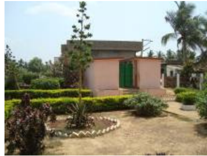
Protected water pond in Pedda Tadepally
