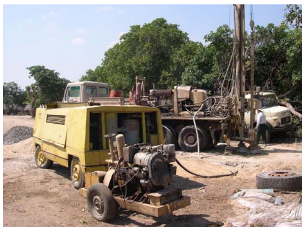
Figure 2 – Large rig mounted on a truck
