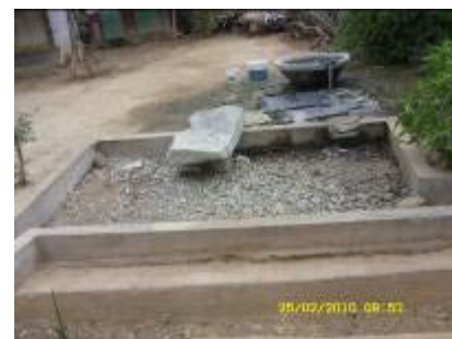
A low cost soak pit at every household and with every water point in Medipally
